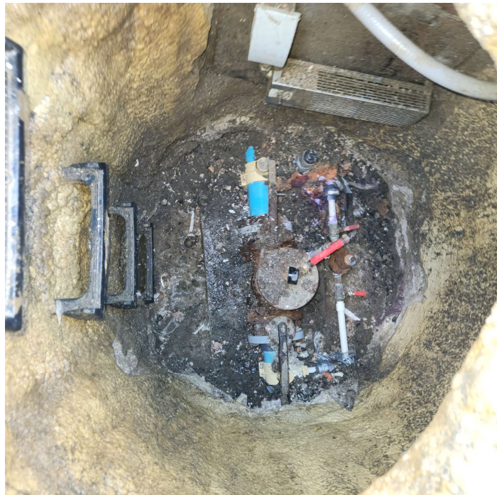
Figure 2-10 - Existing PRV Station
