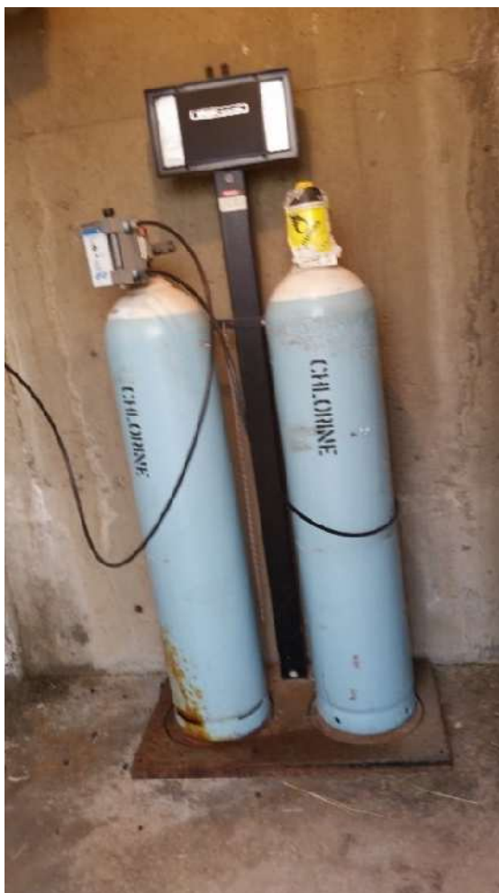
Figure 2-6 - Gas Chlorine Tanks
