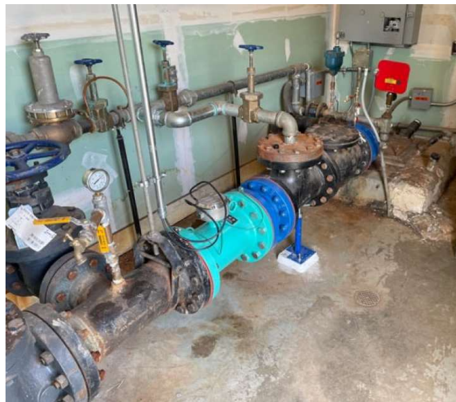
Figure 2-4 - Lower Well House (Inside showing Well 1, and meter)
